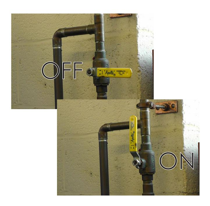
2. Open Machine air valve (on left hand side of machine)
